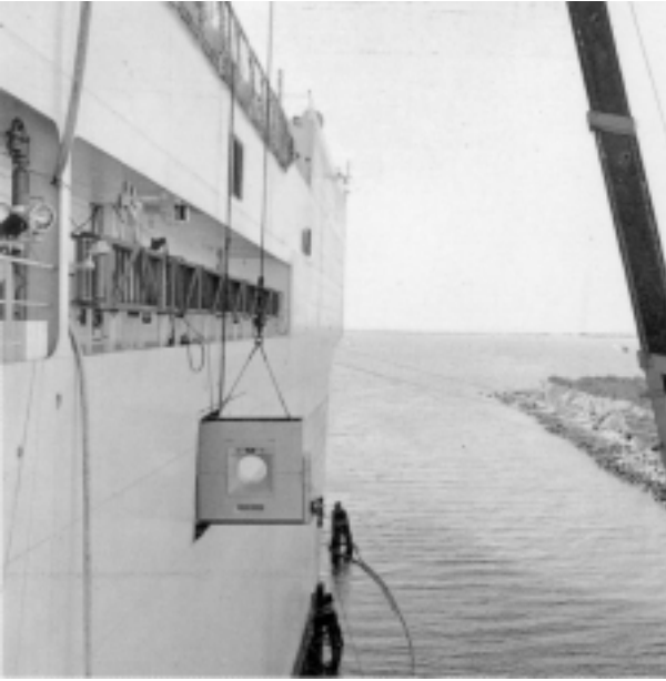
21 Picker CAT 1200 SX CT Scanner, the world's first sea going CT, being installed on the USNS 'Comfort' in San Diego, California in 1988
