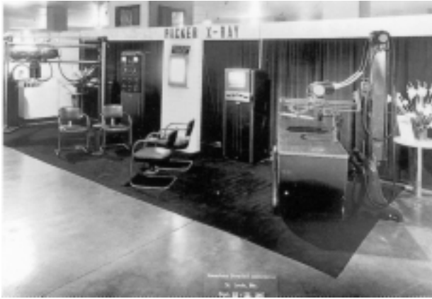
10 Convention, American Hospital Association, St. Louis, Missouri, 1947. The Deep Therapy shockproof unit (220kV) at the extreme left side of the picture was a Picker 'first' in 1933. The design used insulated high voltage cables and insulated tube housings
