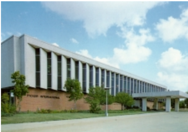
1 The World Headquarters of Picker International, Highland Heights, Ohio – constructed in 1967
